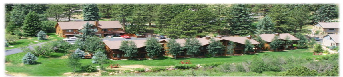
Aspen Winds on Fall River
